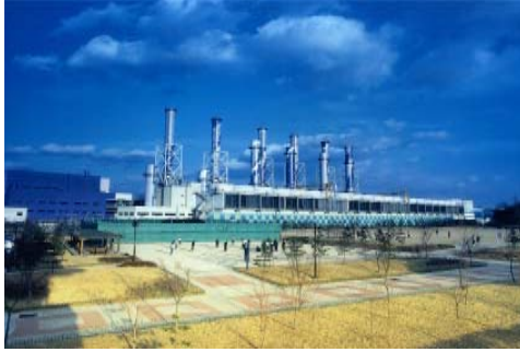
ILSAN Thermal Power Plant
